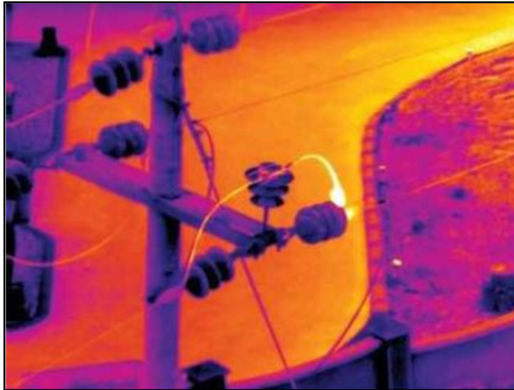
Ferrybridge, 132kV steel pylon circuit & Isle of Wight, wooden pole circuit
