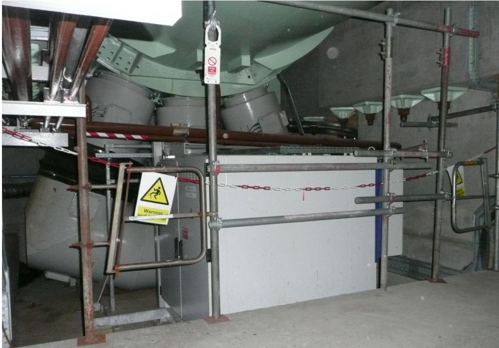
Figure 1 Area around the generator neutral point at Staythorpe Power Station where strong fields were measured
